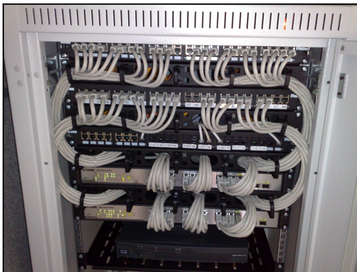
Figure 6.14: Front of the patch panel
